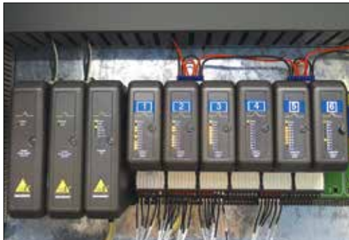
Delta V Fisher-Rosemont Power Supply Systems
