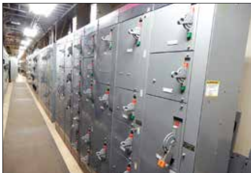
Rockwell Automation AB 2100 Series MCC Sections
