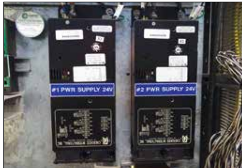
Delta V Fisher-Rosemont Power Supply Systems
